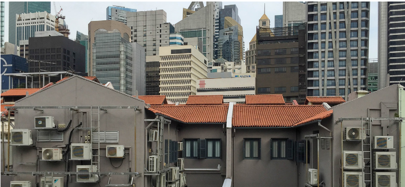
View of outdoor condensing units of air-conditioning systems at a backlane in Singapore, with glass-cladded air-conditioned skyscrapers in the background. (Photo: Chang Jiat Hwee)
