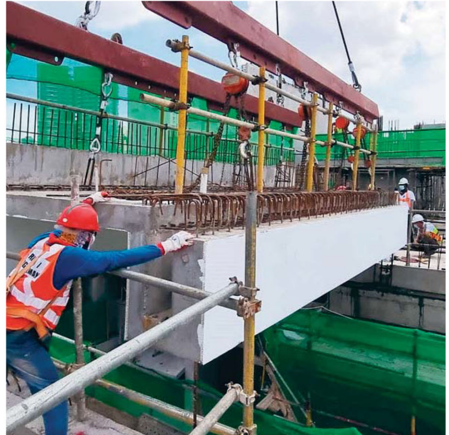
Kwan Yong Construction designed the Integrated Modular Link Bridge, which uses pre-cast parts and pre-installed safety barricades that can be assembled on the ground to minimise risks of falling from height. PHOTO: KWAN YONG CONSTRUCTION
