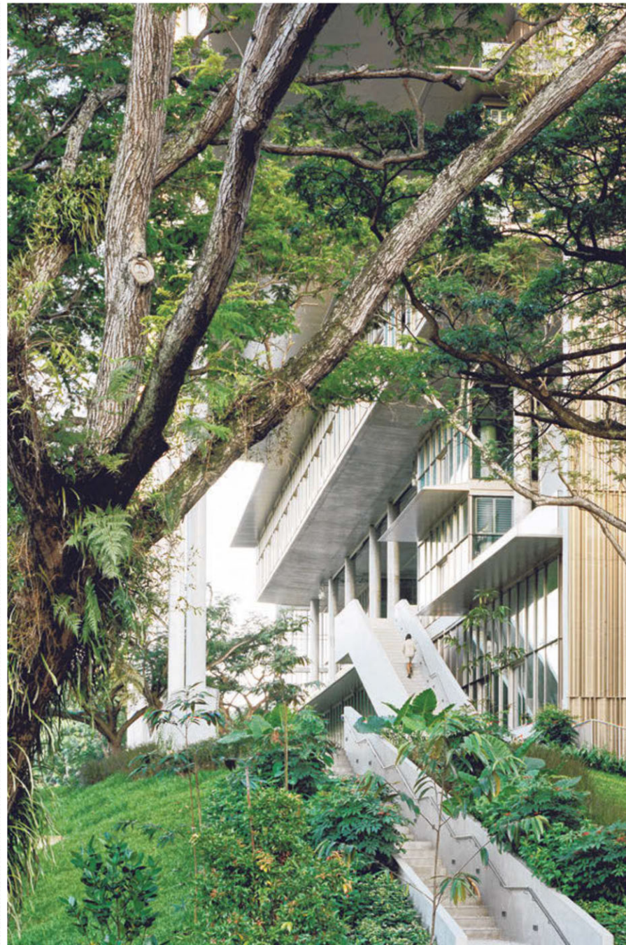
The award-winning energy-efficient zero energy building SDE4 (above) at NUS has sustainable design features holistically integrated into its architecture, such as having more than 1,200 solar photovoltaic panels on its overhanging rooftop to supply renewable energy to meet its energy needs. PHOTO: NATIONAL UNIVERSITY OF SINGAPORE AND SERIE ARCHITECTS
