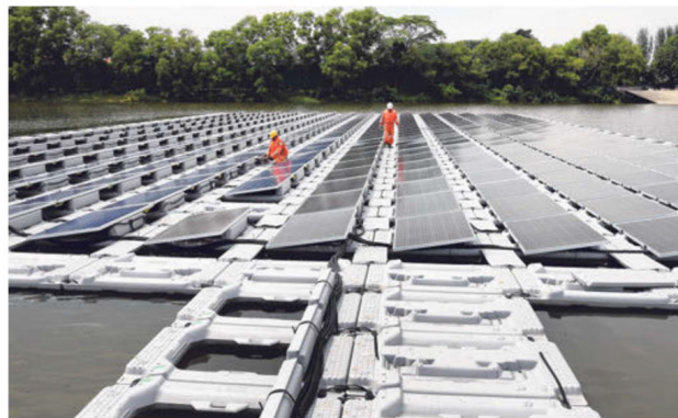
A 2016 photo showing a floating solar photo-voltaic cell test-bed in Tengeh Reservoir in Tuas. Singapore has pledged to peak emissions at 65 million tonnes of carbon dioxide equivalent around 2030. ST FILE PHOTO
