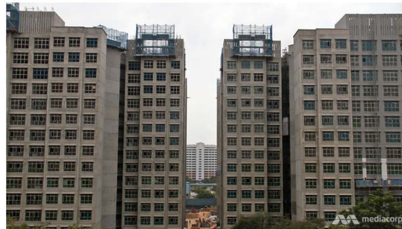
File photo of HDB flats under construction. (Photo: TODAY)
