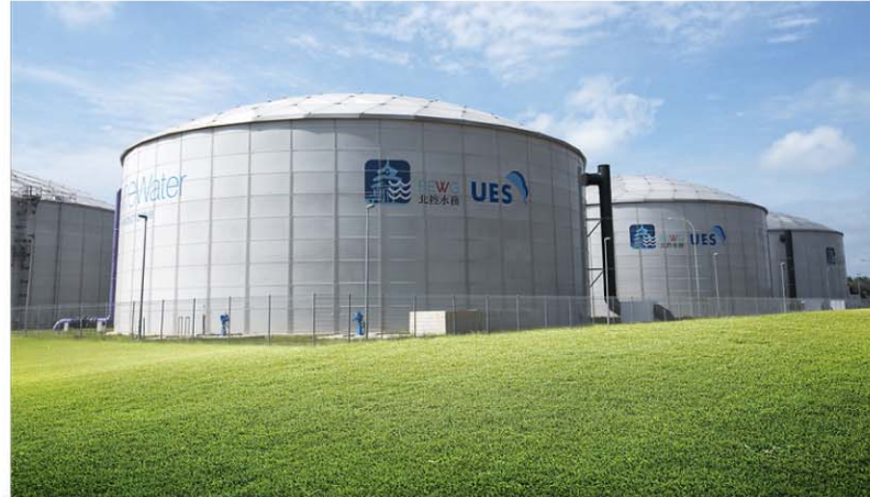
Singapore's fifth NEWater plant located at Changi Water Reclamation Plant. (Photo: PUB)
