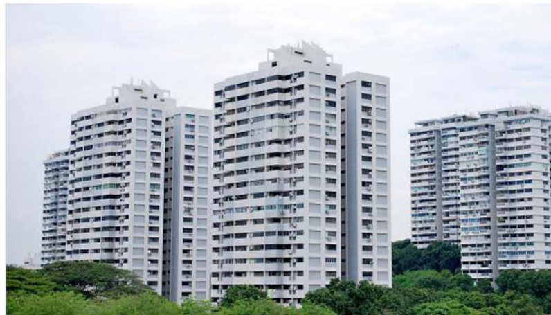
Braddell View (Photo: HDB)
