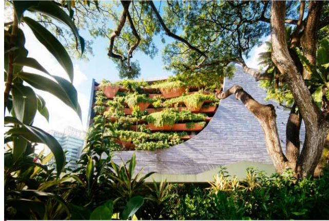
The Lee Kong Chian Natural History Museum has planter boxes integrated into its facade. (Photo: Finbarr Fallon)
