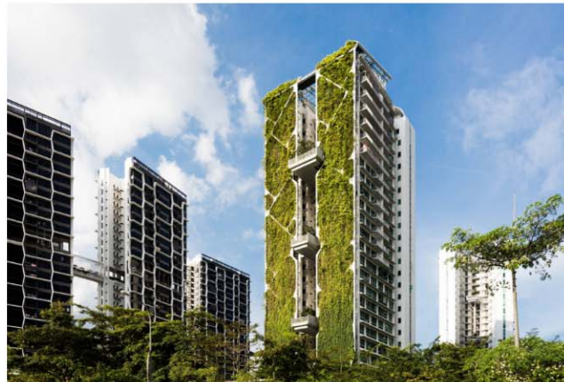
The Tree House condominium in Bukit Panjang has green walls that are designed to reduce ambient temperature. (Photo: Finbarr Fallon)
