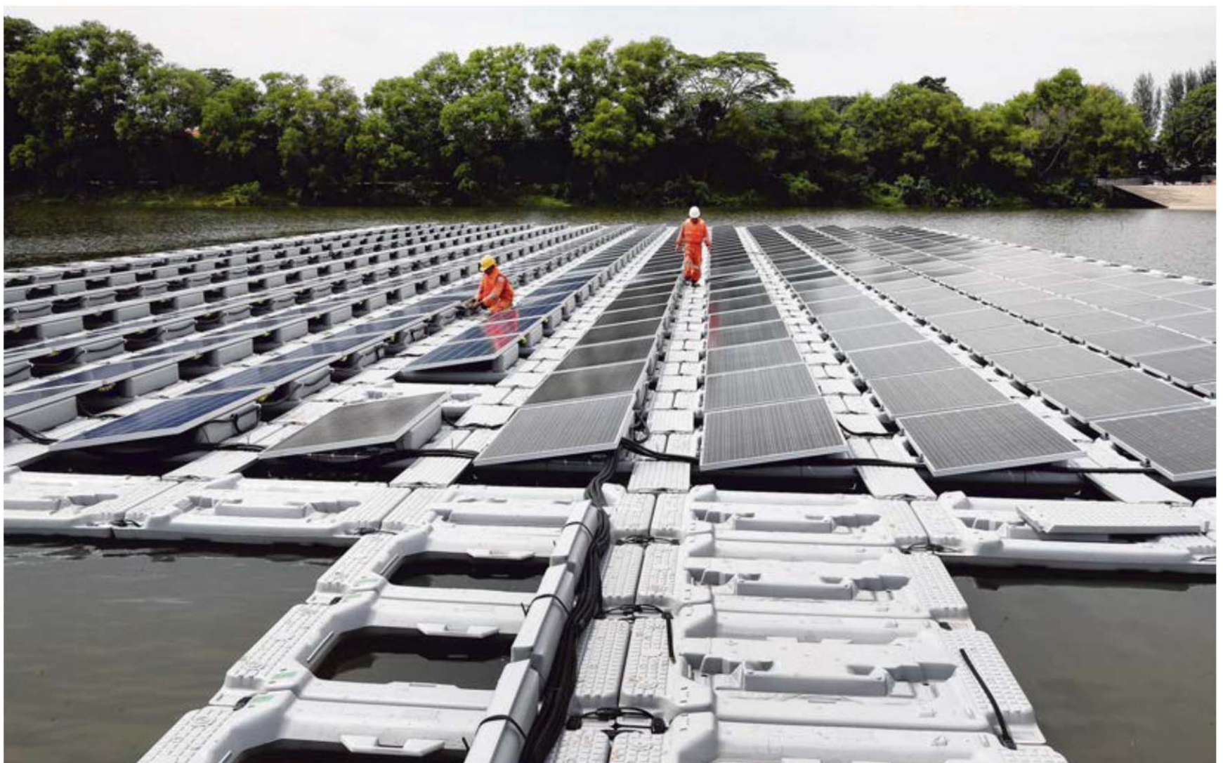
The floating solar panel test bed at Tengeh Reservoir was launched last year to study different photovoltaic systems. Solar energy is important to Singapore since other forms of renewable energy are not as viable here. ST FILE PHOTO
