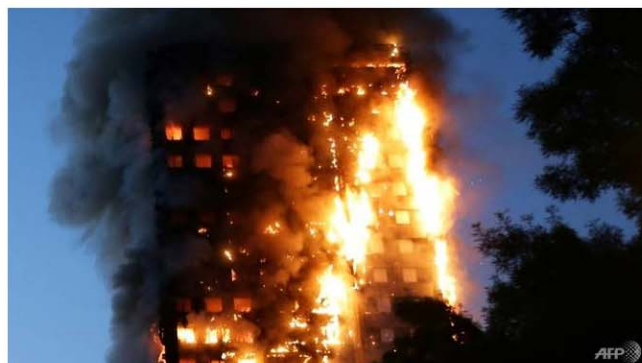
Exterior cladding installed during a recent renovation has been blamed for spreading the fire that consumed London's Grenfell Tower, killing at least 80 people. (Photo: AFP/Daniel Leal-Olivas)
