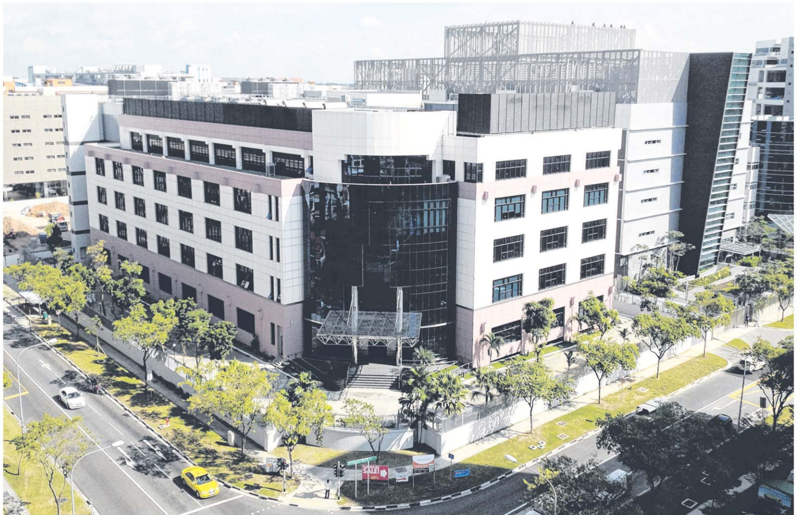
Keppel DigiHub, a data centre owned by Keppel DC REIT, in Serangoon North. The Reit – together with Parkway Life, Soilbuild Business Space, AIMS AMP Capital Industrial and Starhill Global – was among the top five in the new Governance Index For Trusts, the first league table for the 45 Reits and business trusts listed in Singapore. PHOTO: KEPPEL CORPORATION
