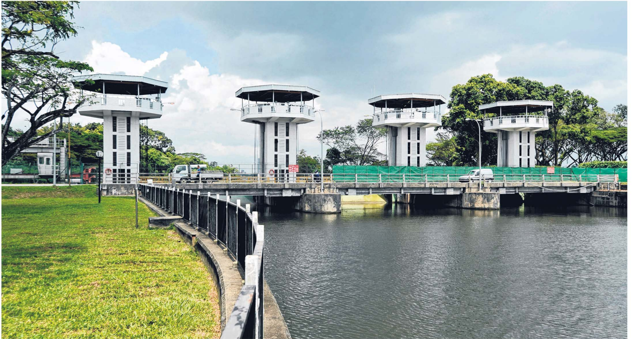
Kranji Water Reclamation Plant, one of five in Singapore designated to turn waste water into potable water, also known as Newater. Singapore aims to be self-sufficient in water by 2060, when water consumption will double from today's level. It will have to accommodate the demands of a growing domestic and non-domestic sector, mainly with Newater and desalinated water. ST FILE PHOTO
