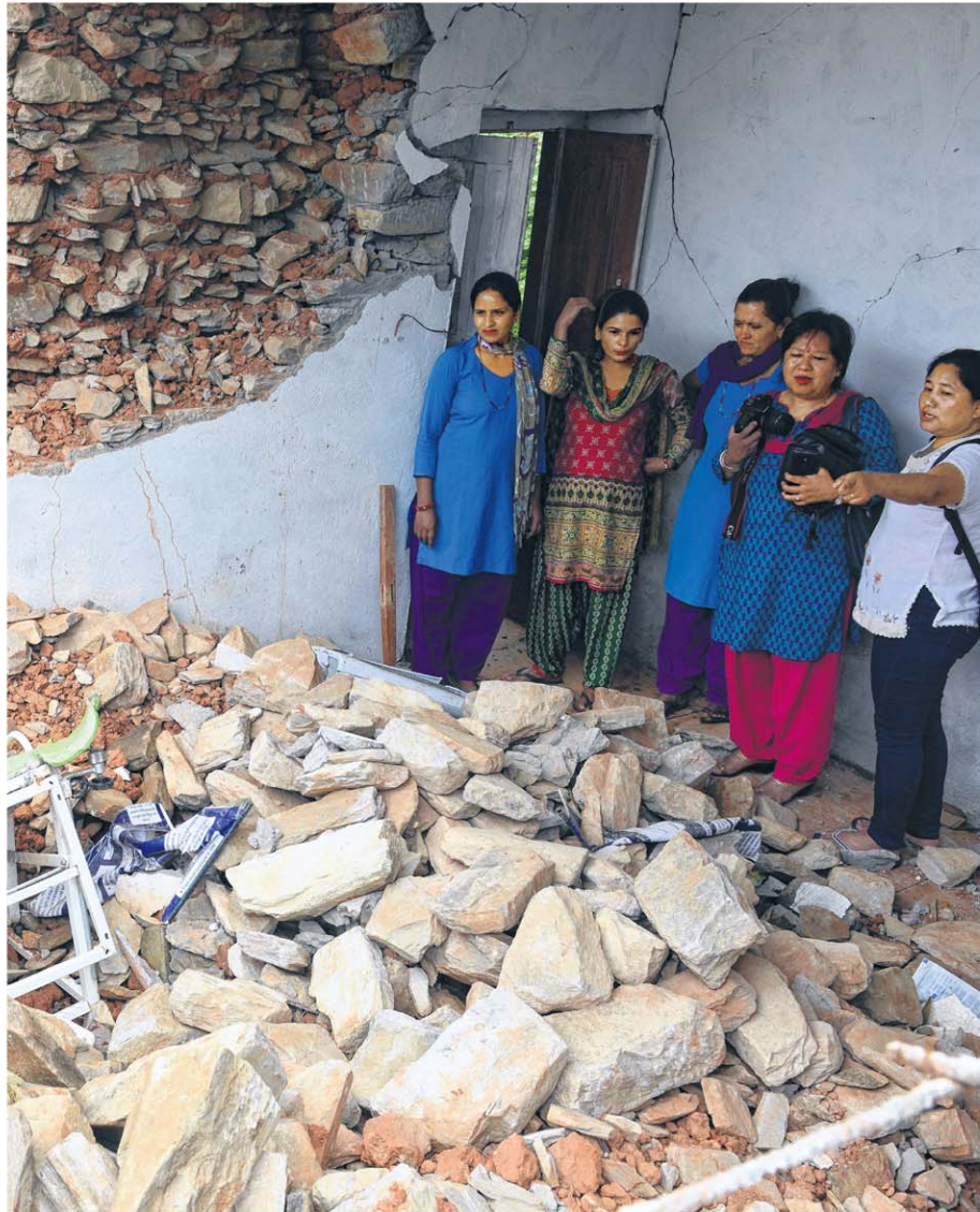
Nepal now faces the arduous task of strengthening institutions, building capacity and improving disaster management policies. PHOTO: AFP
