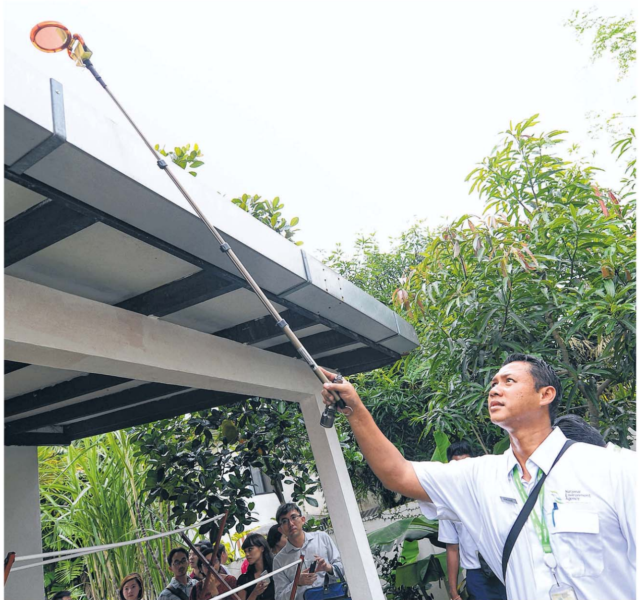
An NEA officer checking the roof of a house for mosquito-breeding sites. Vector control remains a key strategy in the fight against dengue. ST PHOTO: NG SOR LUAN
