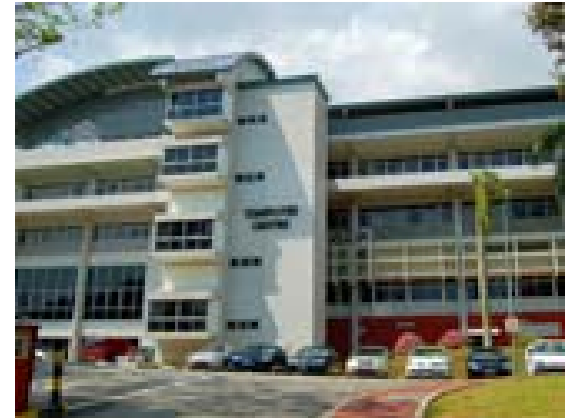
Computer Centre Primary Data Centre
